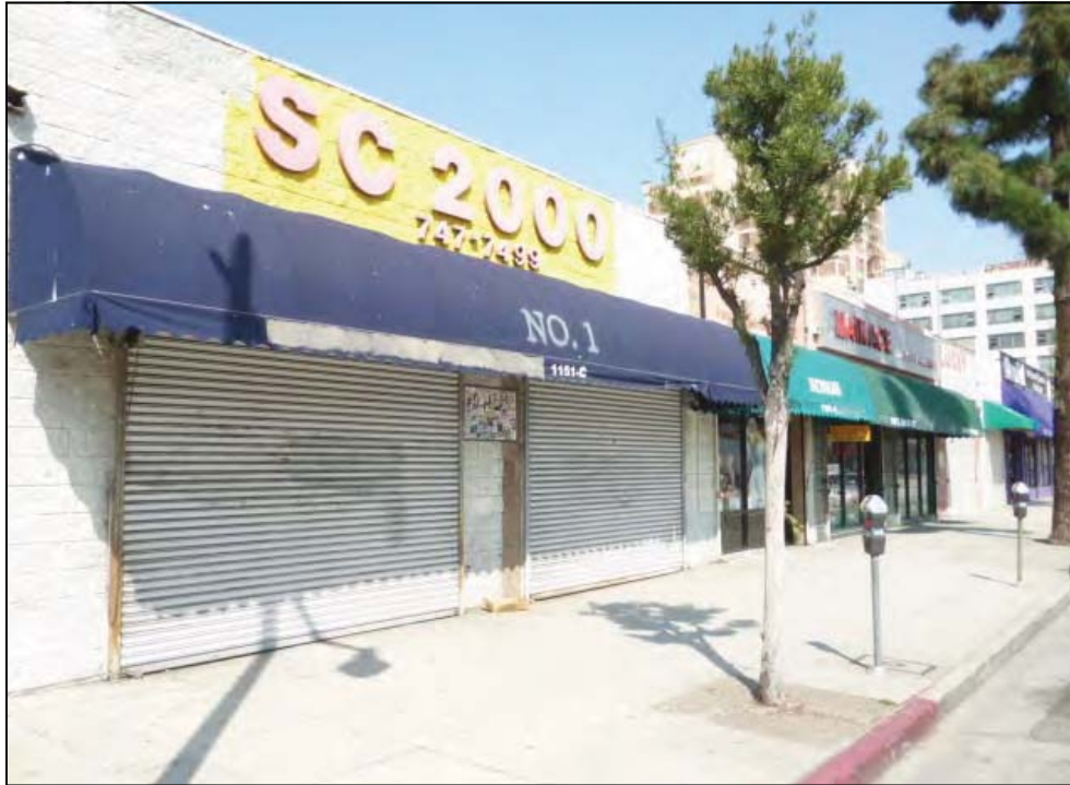
Photo 3: Northeast adjoining property
